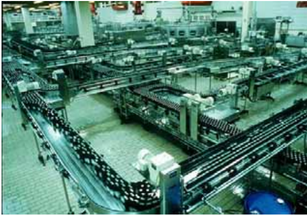
Figure 1. Conveyors of a bottling plant for returnables
